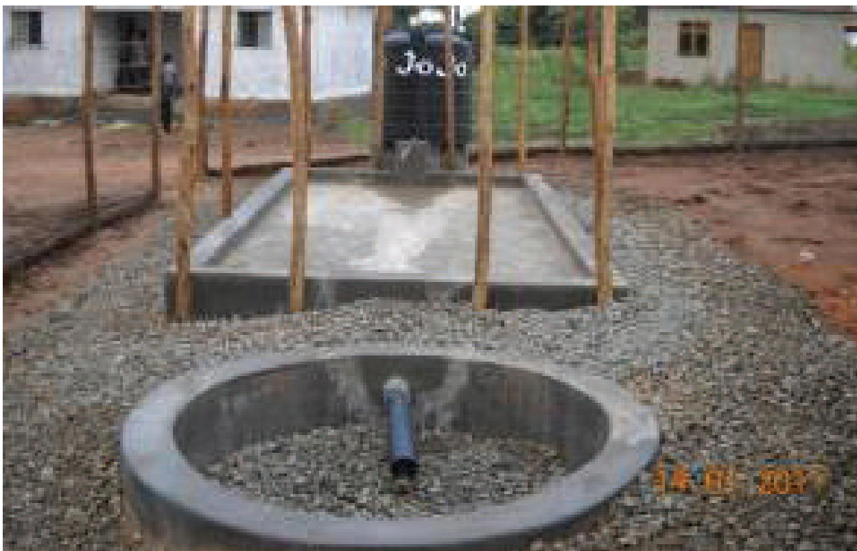
Figure 2: Washing slab connected to effluent Soak Pit.
